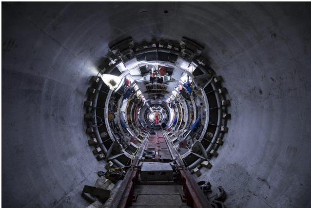
A section of the tunnel in Wandsworth
